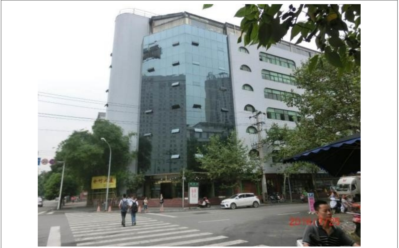
Exterior view and nameplate of the office building
